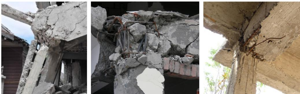
(a) Insufficient anchorage length (b) Unconfined connection (c) Poor coverage
