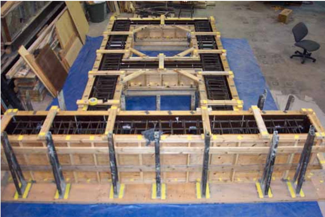
Figure 3.8 Full Steel and Full Formwork Assembly
